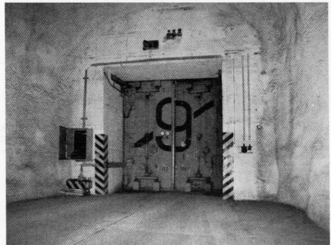
The main blast doors (P on the plan). Photo Tim Robinson
